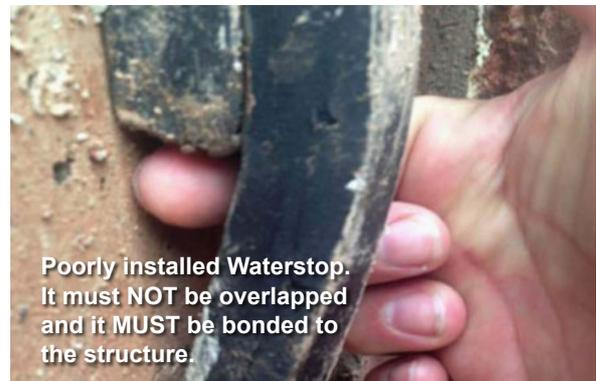
Alternatively, water stops may be cast totally within the site-placed concrete. These are known as internal or centrally placed water stops. Internal water stops will resist the passage of water through a joint from either face. However, they can be more difficult to install and fix, can be dislodged during casting of section and are probably best avoided in domestic basements unless great care is taken and the work properly supervised and inspected.
