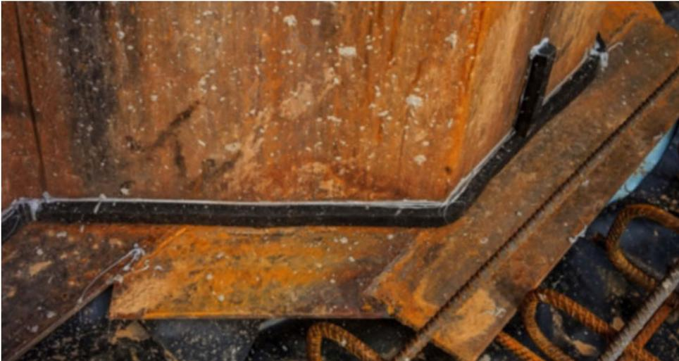
Welded sheet pile wall – floor detail with waterstop.
