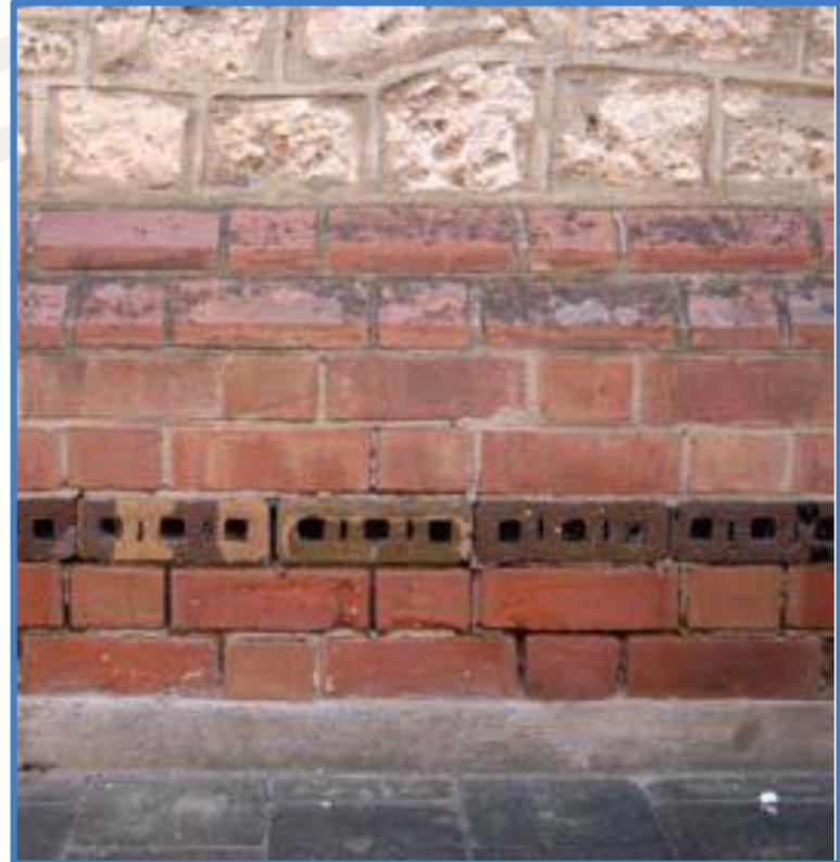
Picture: Salt attack and rising damp - A guide to salt damp in historic and older buildings
